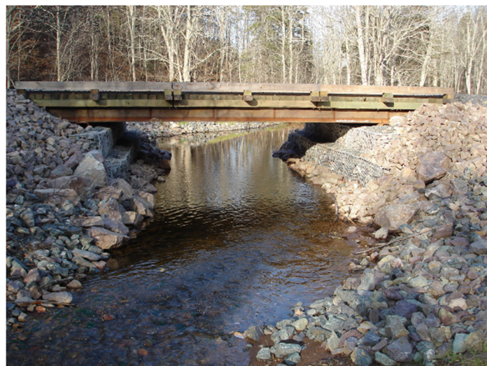
New bridge installation, Paul MacDonald, PHP
